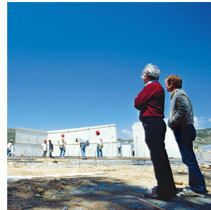
Ed (left) and Richard Hunter look on during construction.
