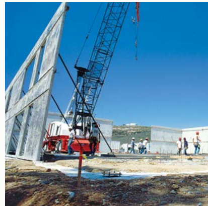
Crew members break ground in 1983 at Hunter corporate headquarters, located at 1940 Diamond Street in San Marcos, California.
